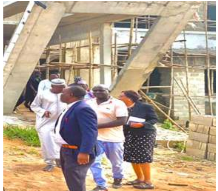
The Vice Chancellor, Prof. Akeem O. Lasisi, other Principal Officers and members of staff during an inspection exercise with one of the Contractors at the University permanent site.
