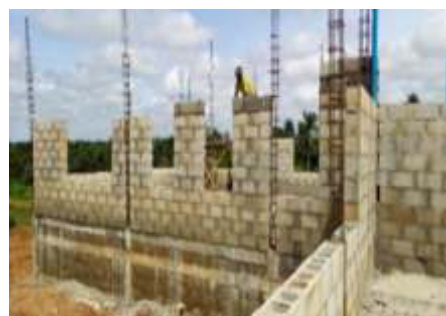
The University Teaching Hospital under construction
