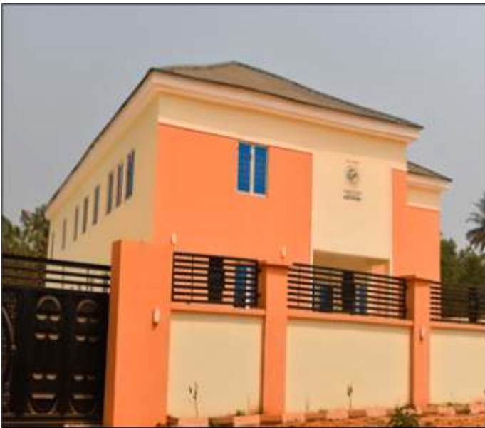
The front view of the University Health Centre
